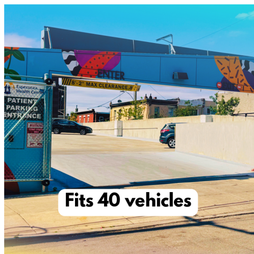
UPPER PARKING LOT #1 ENTRANCE
