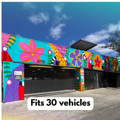
LOWER PARKING LOT #2 ENTRANCE
